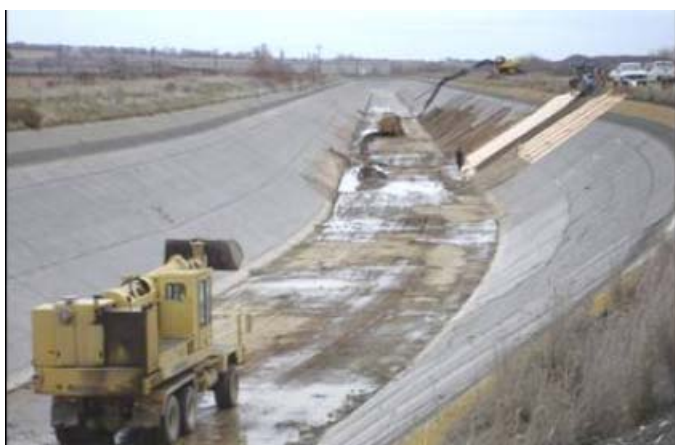
Figure 6 - Irrigation canals like this could be put at risk if aquatic herbicides cannot be used to control vegetation, which can impair the channel's ability to carry water, leading to potential breaching problems.
