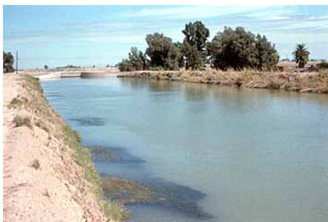
Figure 7 -Aquatic vegetation is beginning to accumulate in patches along the left canal bank of this irrigation delivery system.
