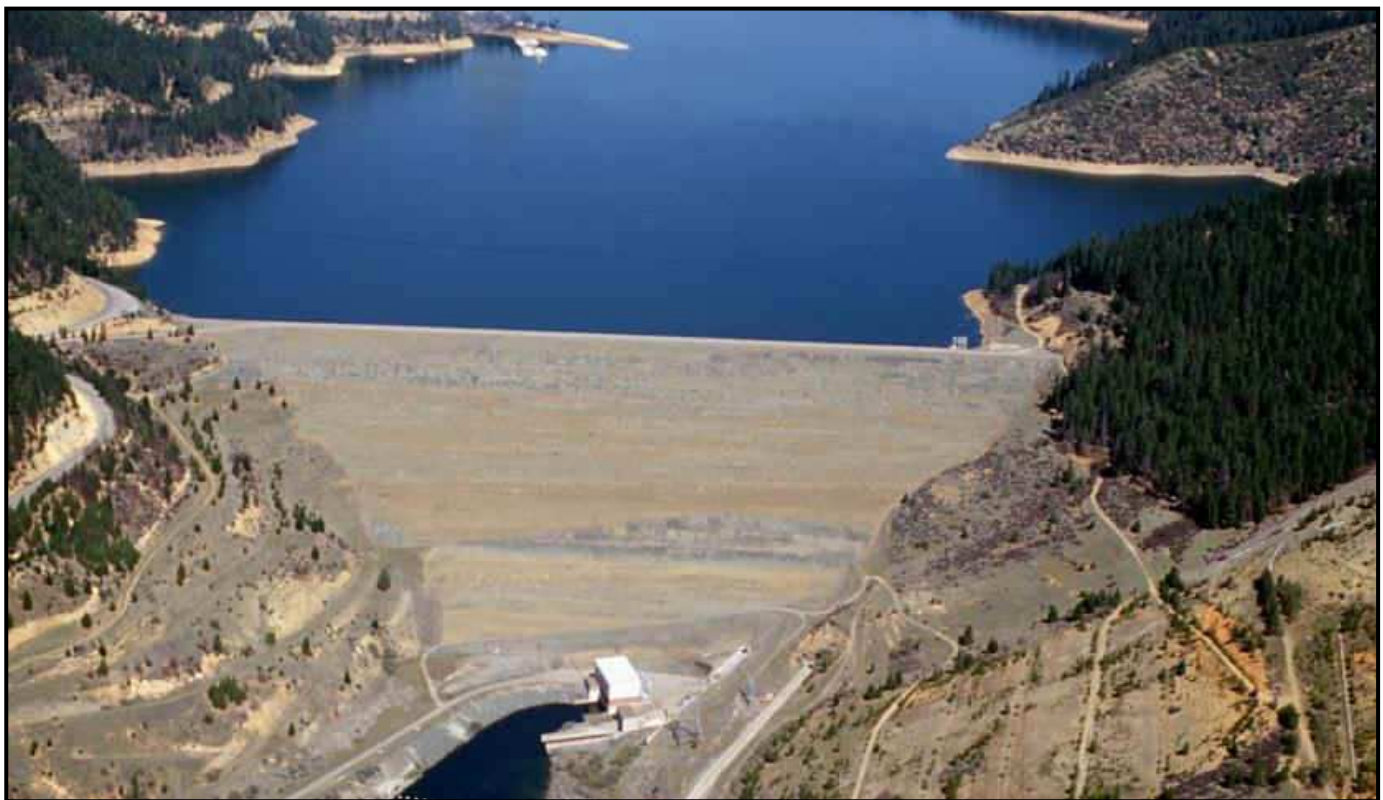
Figure 5: Iron Gate Dam on the Klamath River, one of four dams that will be investigated for possible removal under a new settlement agreement between the United States, California, Oregon, PacifiCorp, counties, farmers, conservation groups, tribes and fishermen. Source: Klamath Bucket Brigade
