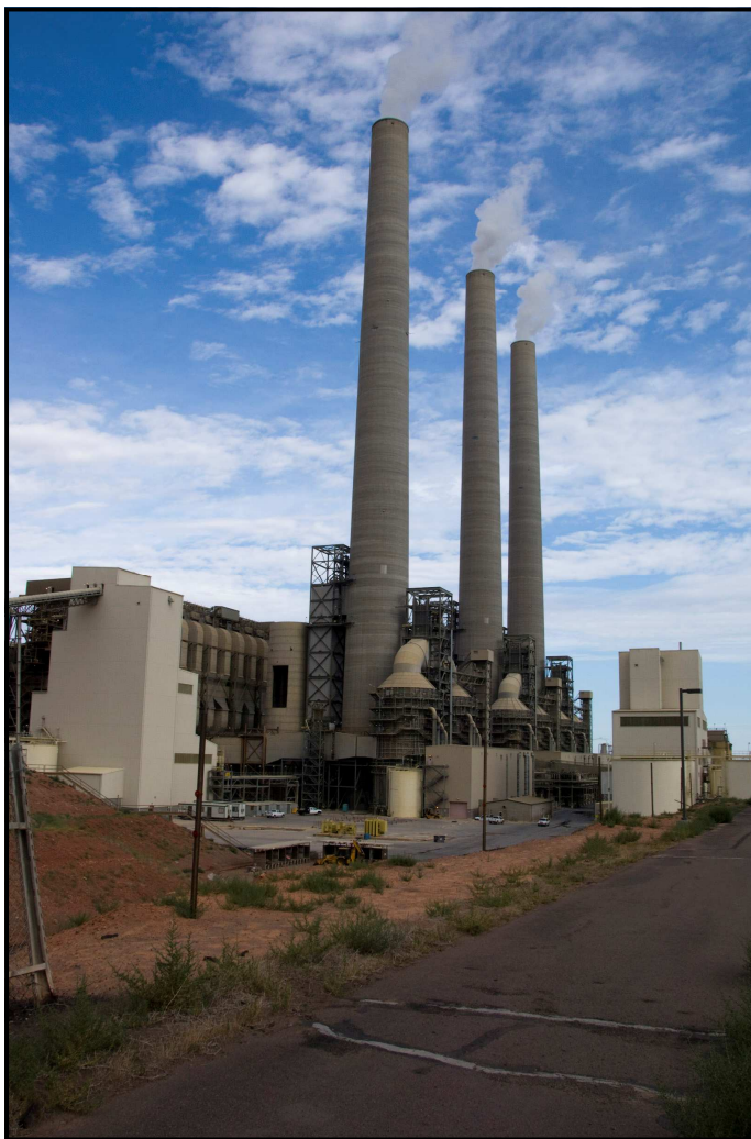
Navajo Generating Station. Source: Central Arizona Project
