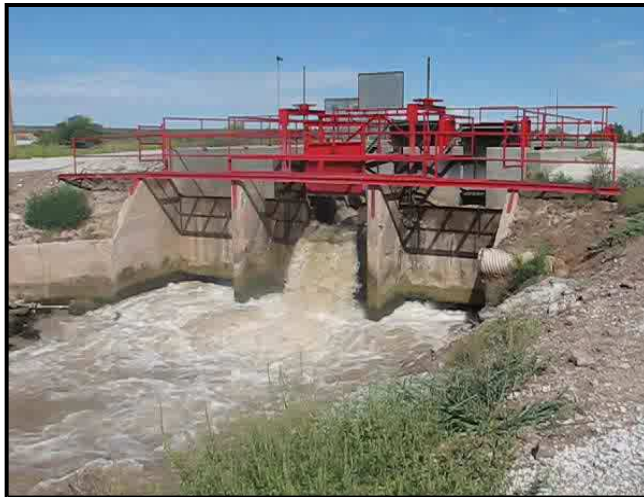
Elephant Butte Irrigation District’s Drop 8 facility flows 300 cubic feet per second and provides an ideal opportunity to install low-head turbines in an existing delivery canal that can produce clean power with no impacts to the environment. Photo Courtesy of EBID.
